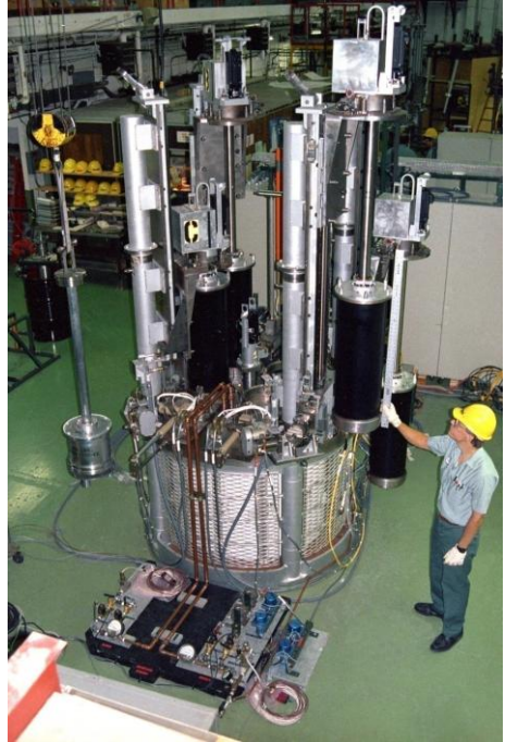
(A) Modular Pyro-Electrorefiner Unit Argonne National Laboratories Chicago
